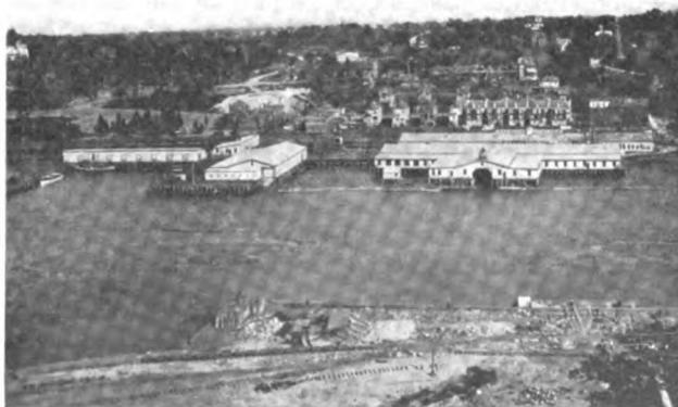
View of the Present Shops
