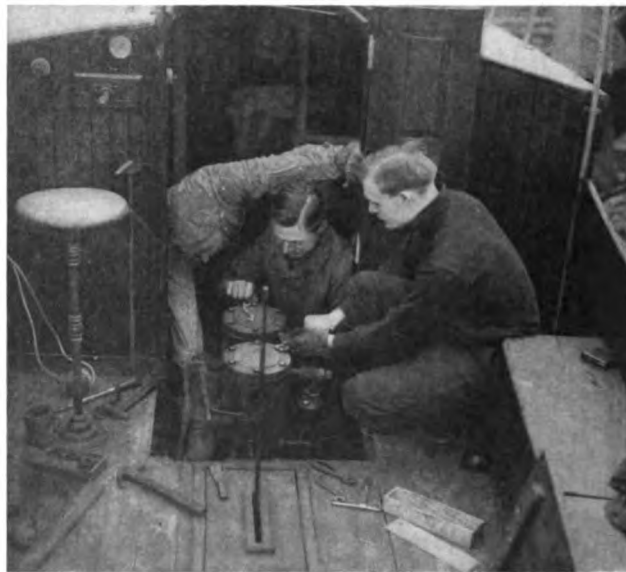
If Your Engine Is Installed Where It Is Difficult to Get at, Take It Out and Mount It on Trestles Alongside
