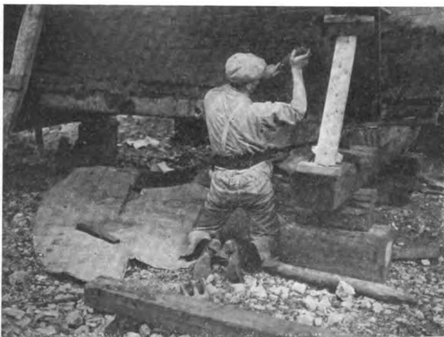
Cleaning Off the Bottom with a Wire Brush
