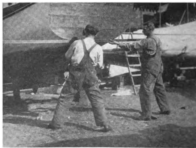
Raising the Water-Line
